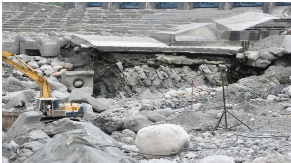
Figure 14. Outcrops of brittle fractures in the zones of shear banding and shear texturing in the riverbed downstream of the Shigang Weir.
