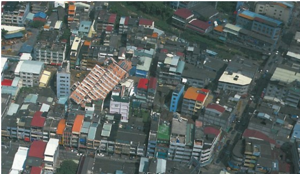
Figure 16. Tilting failure of the Wangchao Building during the 921 earthquake (Lian, 1999).
